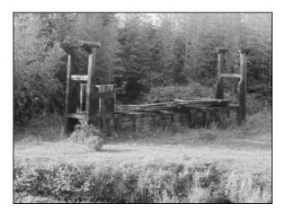
Figure 5. A "trunk" used for field irrigation. Note the swing gates located at either end. Photograph by Charles F. Kovacik.
